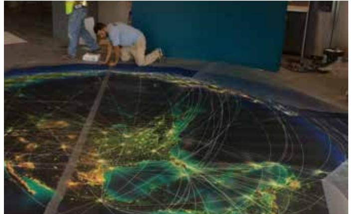
LSI Custom Printed floors are flexible and will handle easily when cutting and fitting. This characteristic enables the installer to fit the material using freehand knifing techniques. Plan your layout before cutting material. Measure and square up area to be installed. If the job site is complex and requires a precise fit, use pattern-scribing techniques. LSI Custom Printed floors may also be fit using direct scribing techniques.
